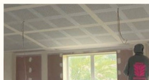
PLASTERBOARD STOPPING
